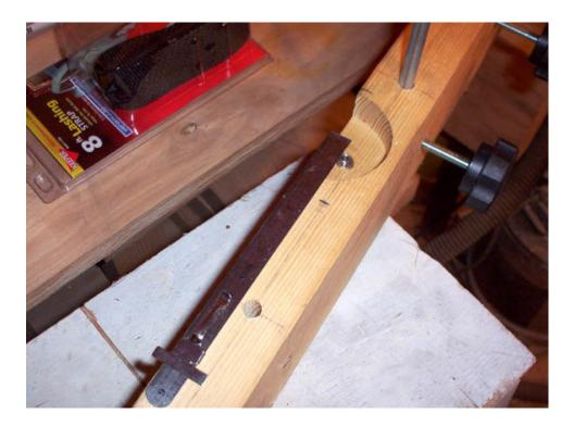
The eyebolt I'll be using is around 8" long and there will need to be a 1/4" hole drilled all the way through the 2x4.
